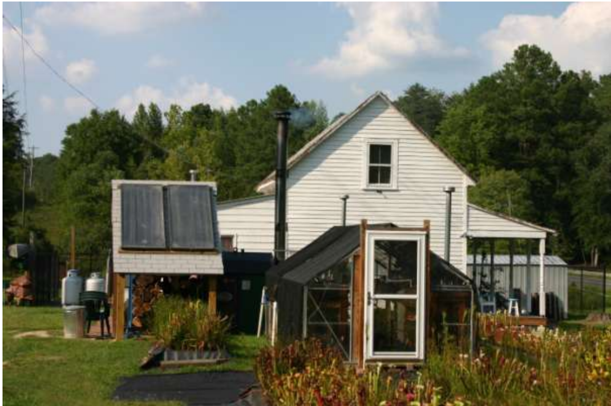
Figure 7. Outside wood furnace and hot water solar panels provide domestic hot water and heat facilities at Meadowview.
